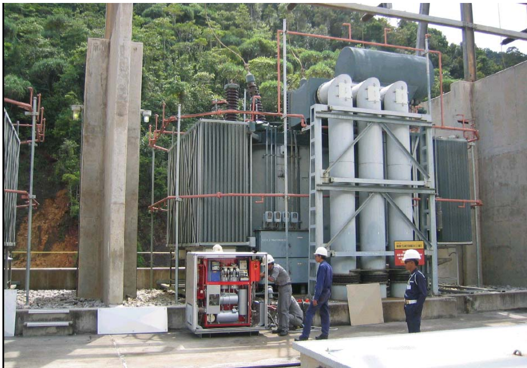
Germany: 250 MVA Transformer
