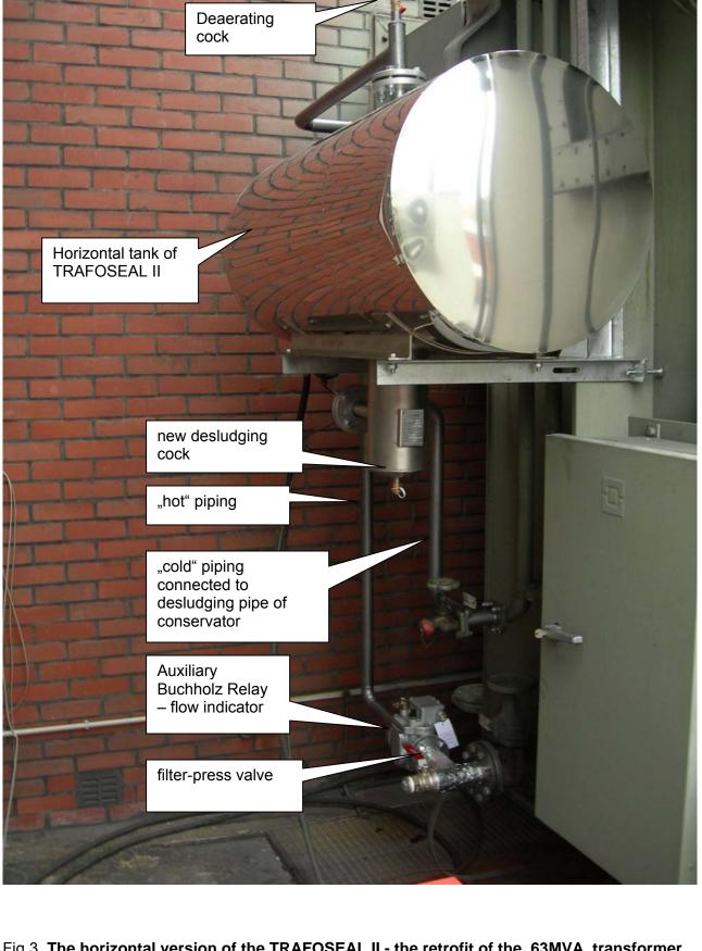
Fig.3 The horizontal version of the TRAFOSEAL II - the retrofit of the 63MVA transformer.
