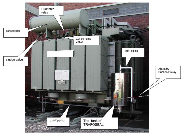
Fig. 2 The standard retrofit of the 17MVA furnace transformer using the vertical TRAFOSEAL tank
